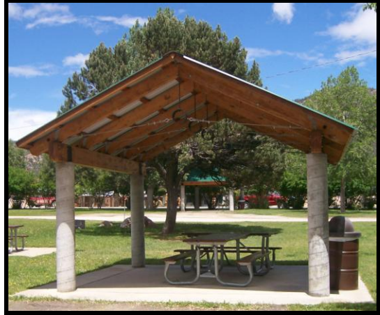
Photo 6: Example of permanent shade structure
