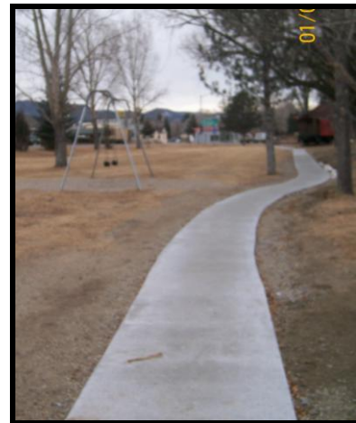
Photo 12 : Constructed path at McPhelemy
