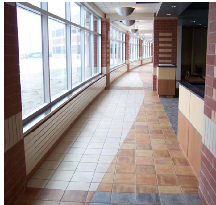
Figure 2: Runtal Baseboard Radiation Installation
