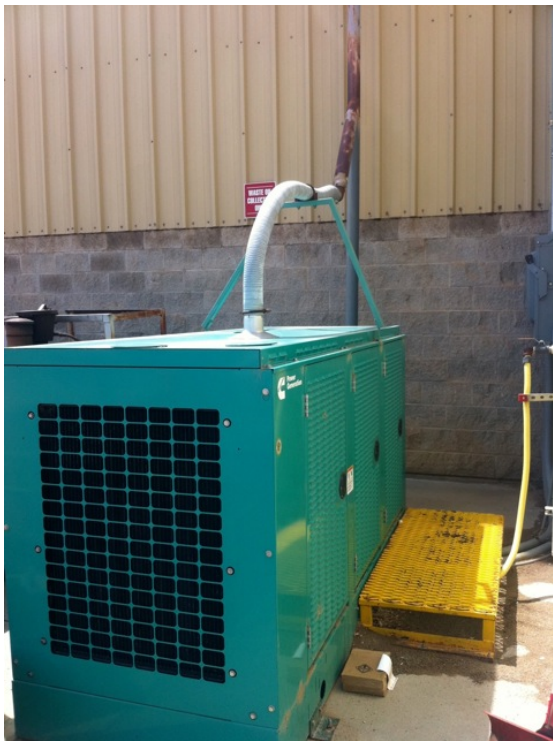
Figure 4 Diesel generator providing back-up power for City of Cortez' CNL
