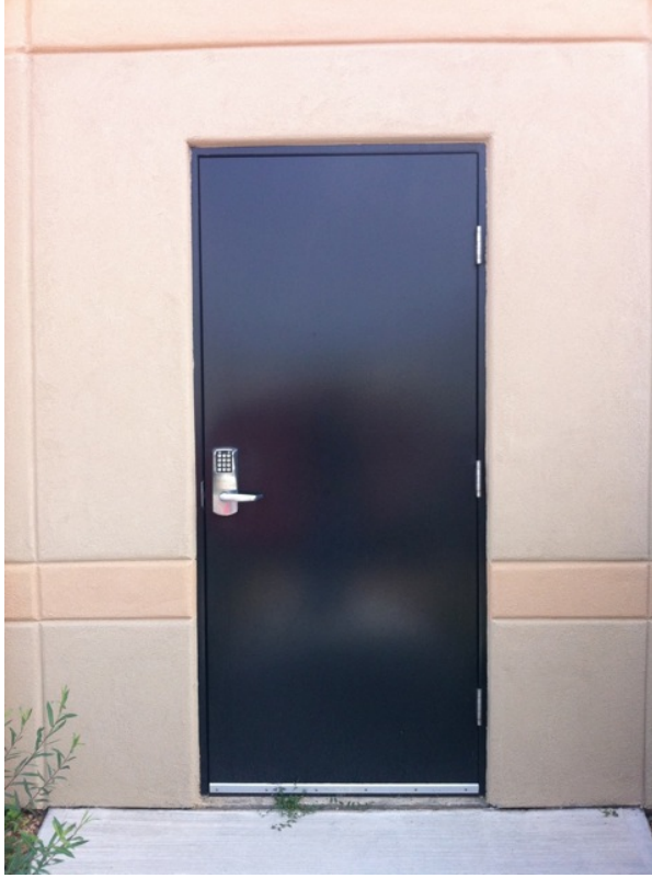
Figure 7 Secure entrance to the CNL ensures security and reliability
