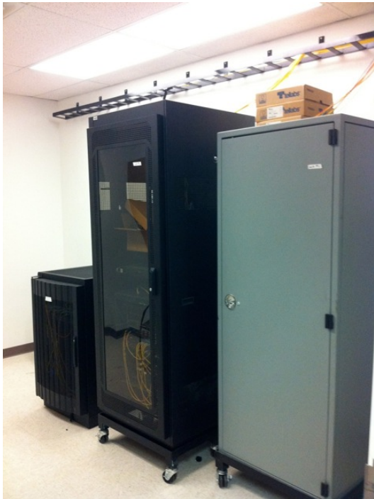
Figure 6 Rack space for Middle and Last Mile service provider switching and routing equipment in Cortez CNL
