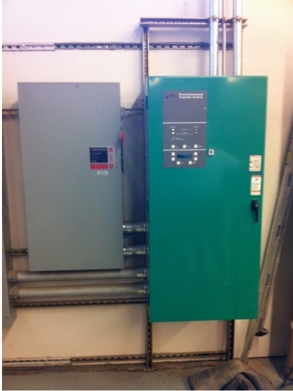
Figure 5 Uninterruptible Power supply (UPS) for Cortez CNL
